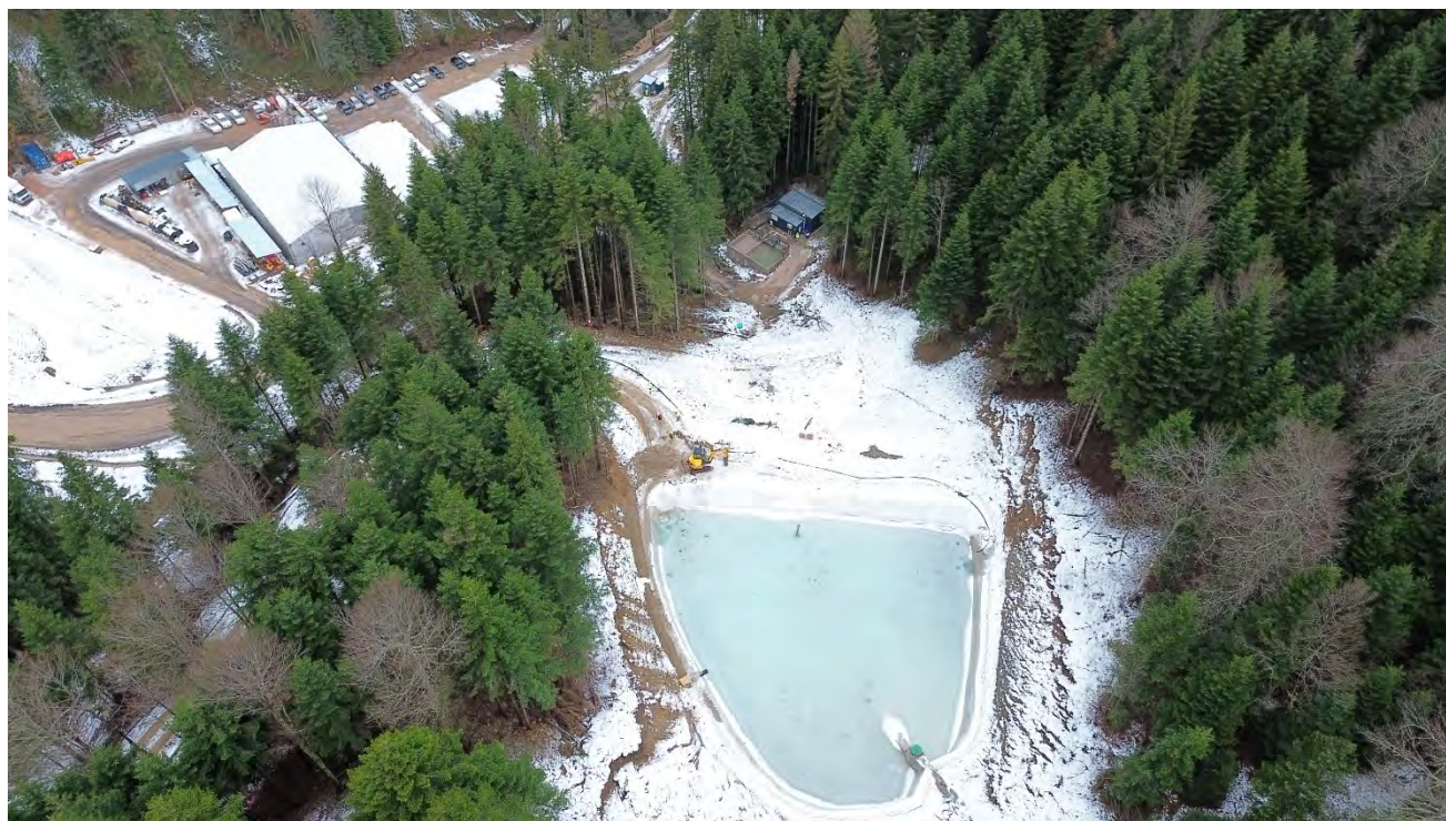
Figure 7: Water Treatment Plant, December 2023
