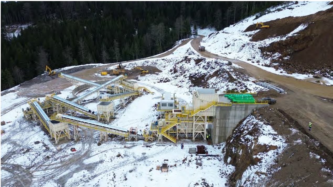
Figure 8: Crusher Plant, December 2023
