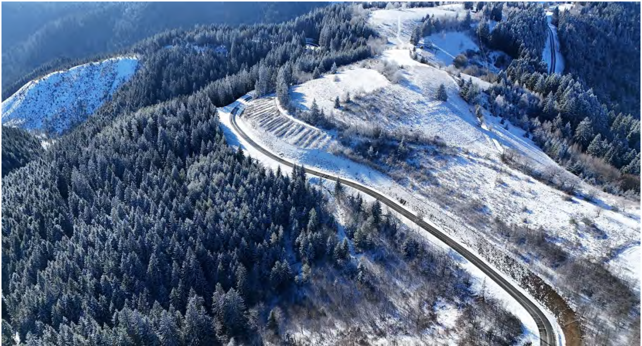
Figure 14: Aerial view of the completed road, December 2023
